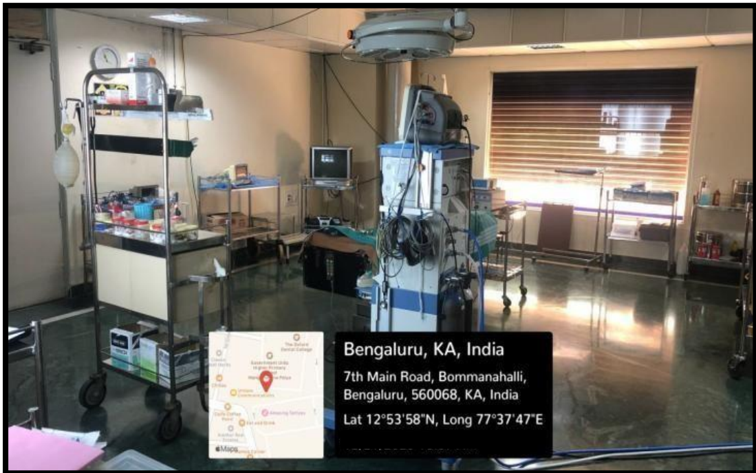
Minor Operation Theatre
