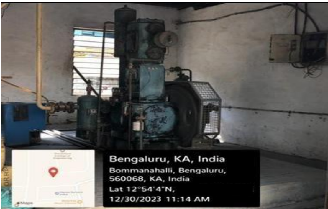
Centralized Compressor for Dental Departments
